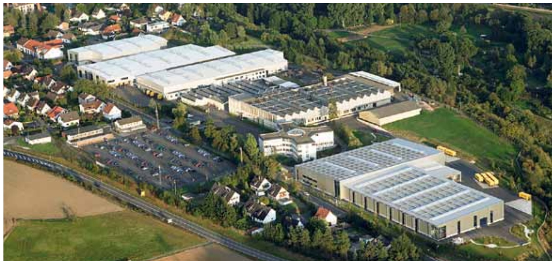
Plant at Meisenheim
